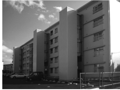
Fig. 2 Residential Building with Added Elevator Towers
