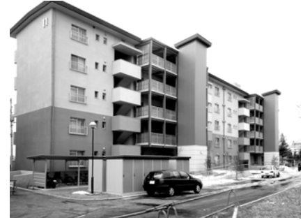
Fig. 3 Residential Building with Added Access Corridors
