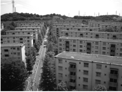
Fig. 1 Housing Estate Built in the Mass-housing Era
